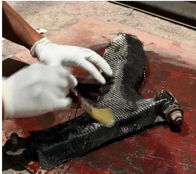
Fig. Carbon fiber reinforcement using resin solution
